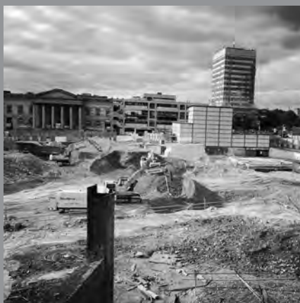
Elephant demolition, October 2021.
